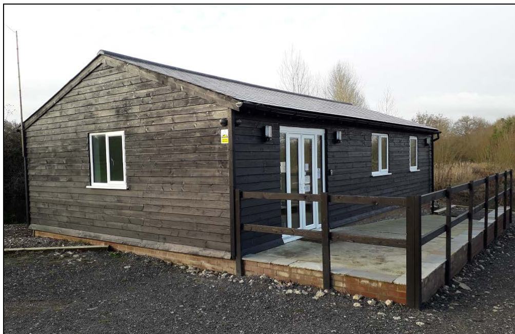
Figure 6 – Existing amenity block
